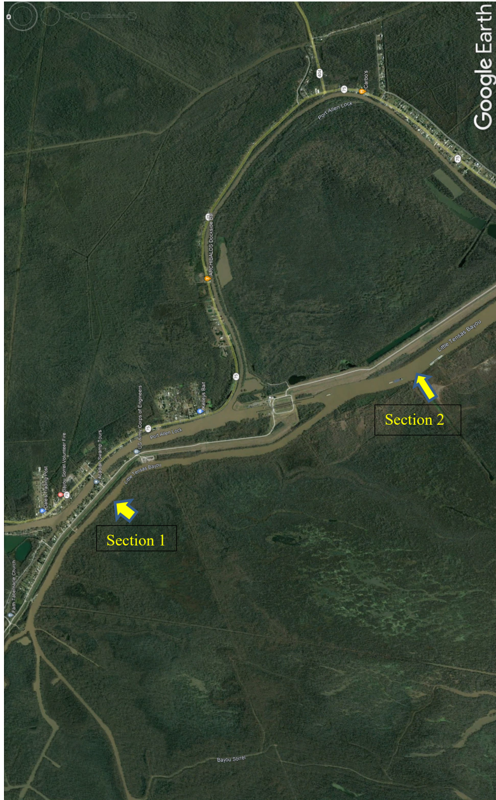
Figure 1. Google Earth Image showing the very distinct difference in the widths of channels as marked.
