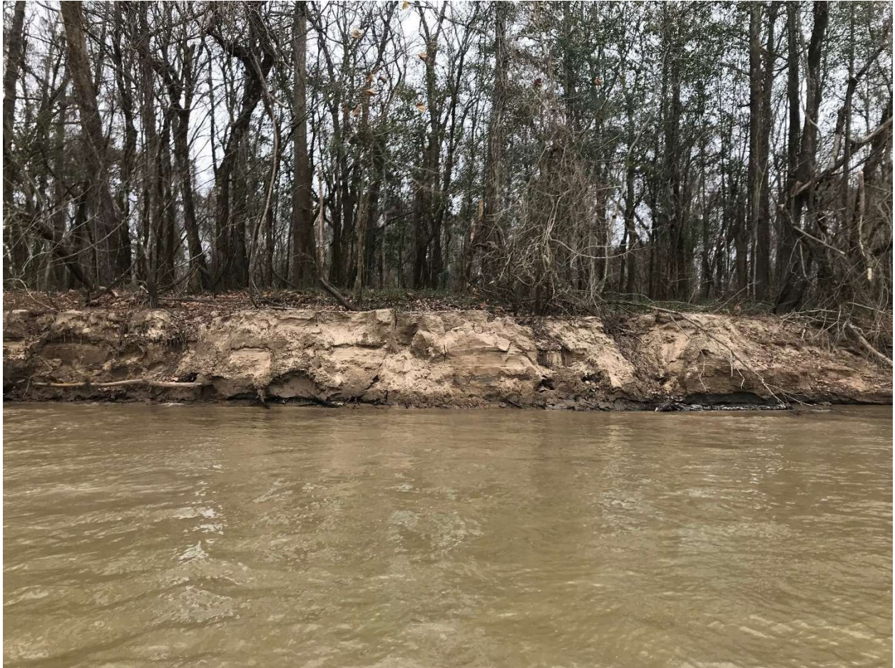
Figure 12b. Photograph of the levees along Bayou Sorrel Diversion Channel inside of the Atchafalaya Floodway. Bayou stage was +4.0 feet on 7 th January 2018 and levees about 7.0 feet above stage. Approximately same latitude as Figure 12a.
