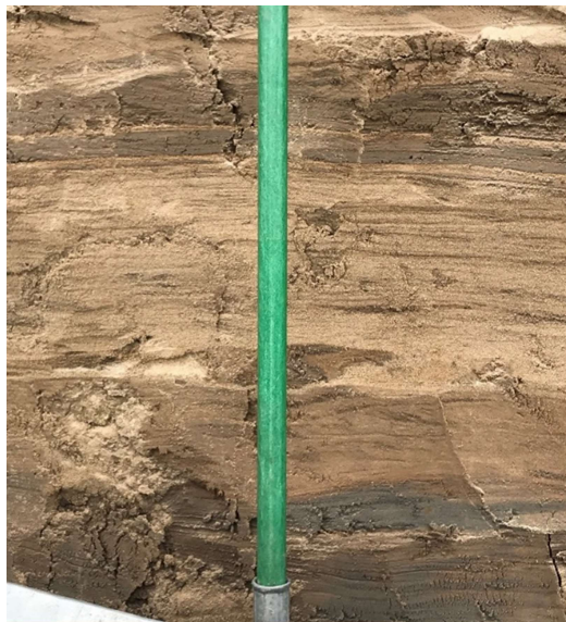
Figure 5. Suspended sediment deposits in the levee along the Bayou Sorrel channel within floodway showing different sedimentation cycles. Spade handle for scale.
